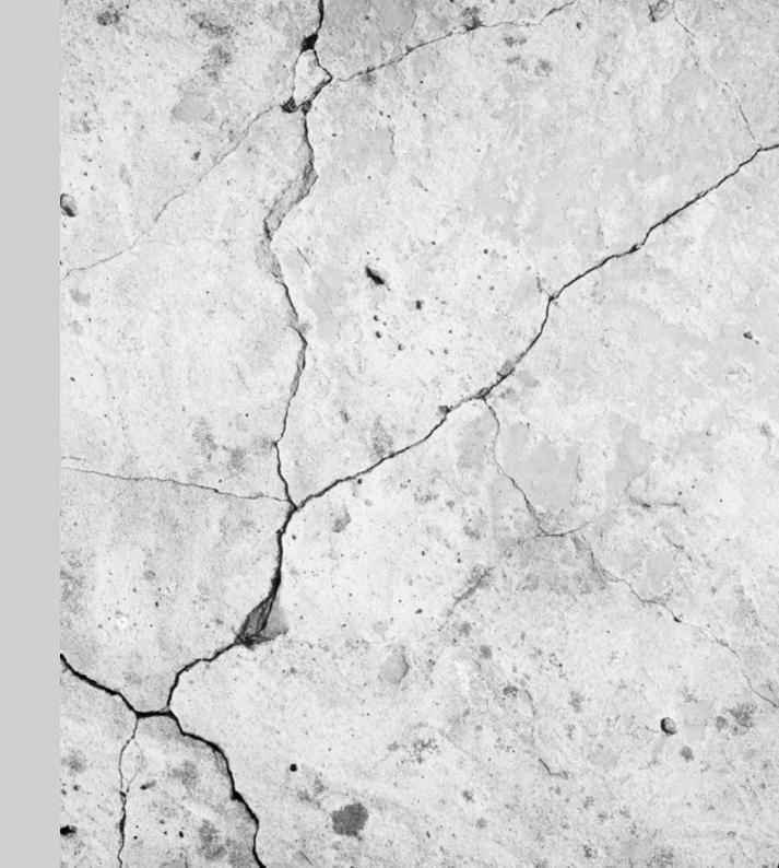
A certain amount of cracking could have occurred because of drying shrinkage and usually this isn't a significant problem (although it should be regularly checked to make sure it doesn't get worse).
