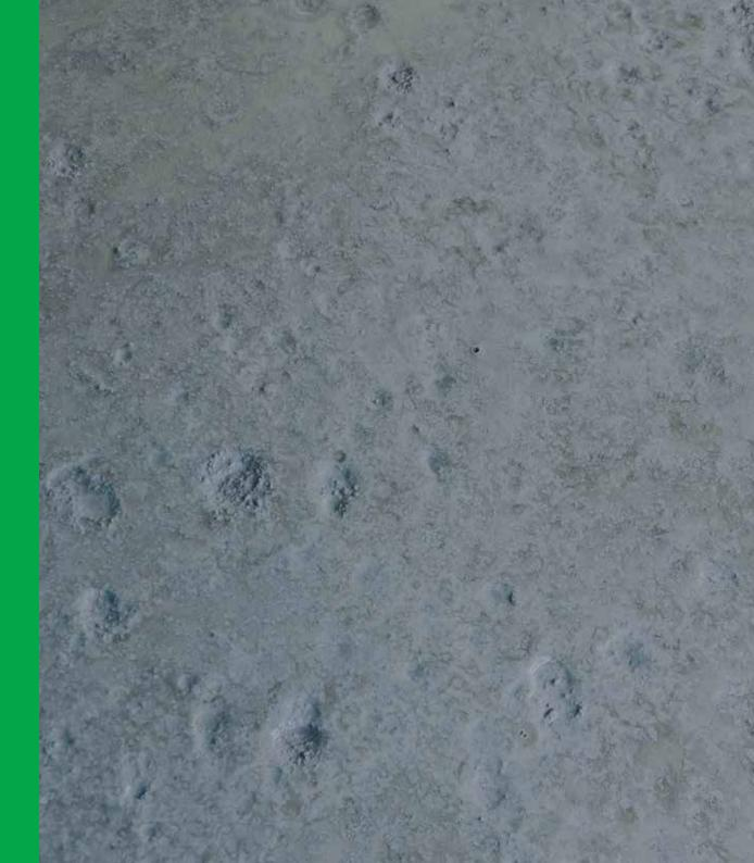
There are several reasons for this, which can range from external water getting into the screed, condensation, spillages and leaks or applying the finish before the screed has dried out.
