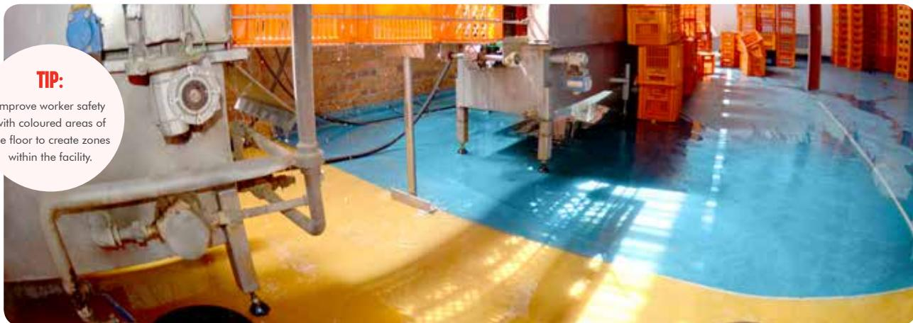
The non-porous and difficult to penetrate nature of polyurethane helps to avoid bacterial contamination as pathogens cannot seep into the floor and are much easier to remove during cleaning. This solution is better than epoxy alternatives at resisting bacterial excretion on the floor, which is especially beneficial in areas of the dairy that are prone to contact with excessive amounts of dung.
