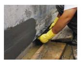
$\blacksquare$  • Apply a first coat of VANDEX BB 75 E (3 kg/m², 1.5 mm, mixing instructions as per Data Sheet VANDEX BB 75 E), at least 1 cm beyond the VANDEX CONSTRUCTION JOINT TAPE.
