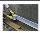
**3.** Overcoat VANDEX CONSTRUCTION JOINT TAPE with a second coat of VANDEX BB 75 E ( $2 \text{ kg/m}^2$ , 1 mm) and smooth the surface with damp brush.
